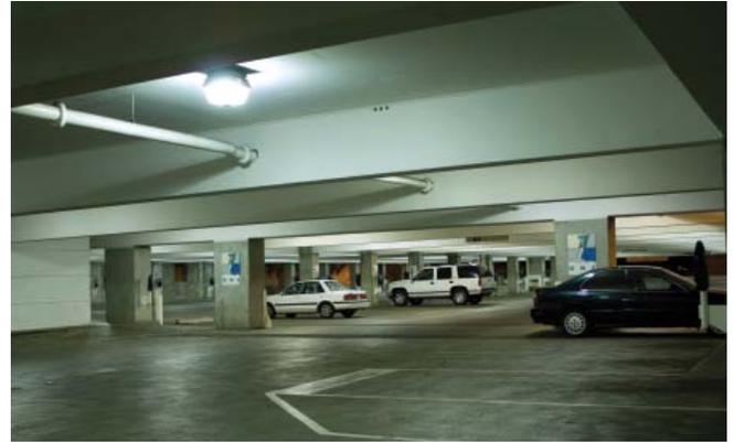
been retrofitted with bi-level induction parking luminaires and a Wireless Interface for Photosensor and Motion Sensor system (WIPAM).
