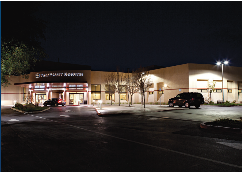
LED luminaires with state-of-the-art lighting controls light the walkways, parking lots, and emergency vehicle routes at NorthBay VacaValley Hospital
