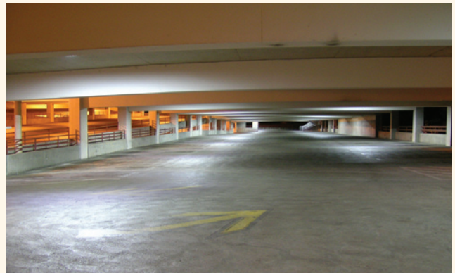
FIGURE 1: POST-RETROFIT BI-LEVEL LED LUMINAIRES
