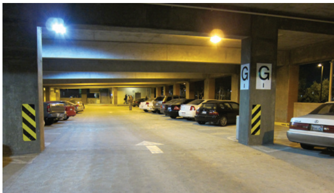
FIGURE 4: POST-RETROFIT BI-LEVEL LED LUMINAIRES
