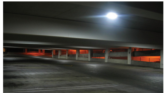
FIGURE 2: POST-RETROFIT BI-LEVEL LED LUMINAIRES
