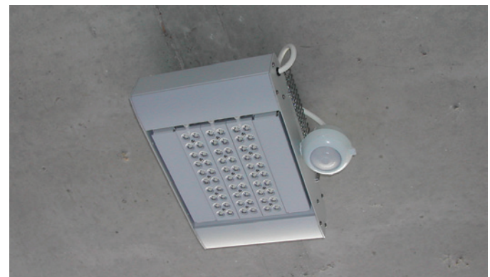
FIGURE 3: BETALED THE EDGE PARKING STRUCTURE LUMINAIRE
