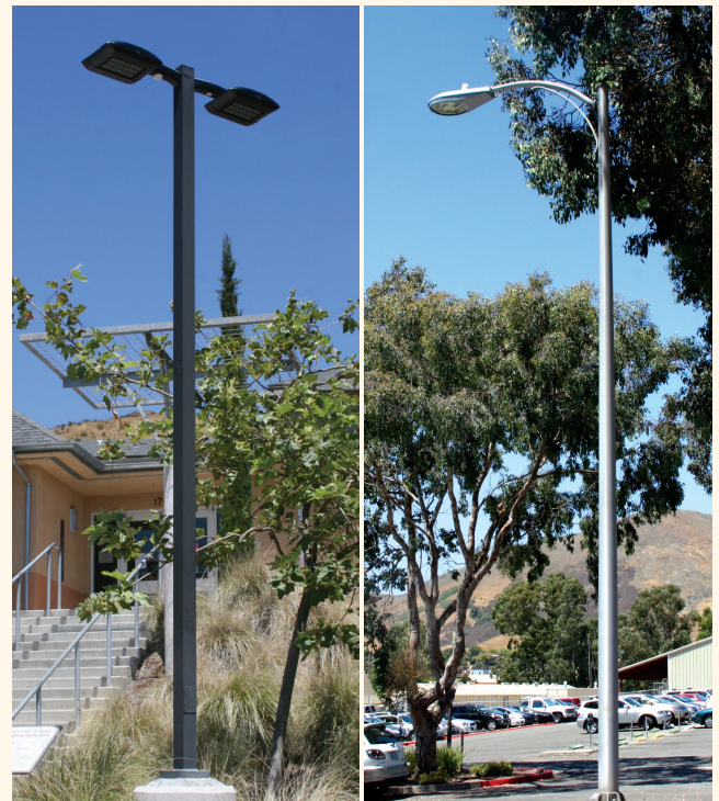
FIGURE 1: BI-LEVEL STREET AND PARKING AREA LUMINAIRES
