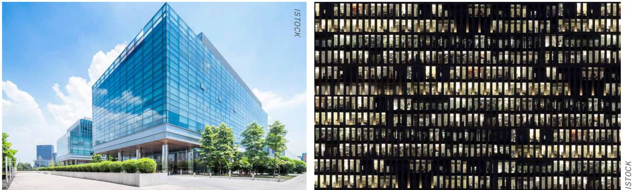
**FIGURE 42** Reflective glazings prevent view of interiors from the outside during the day, as the reflected radiation is significantly higher than that transmitted from the interior light levels. However, they allow a clear view of interiors during the night when the electric lights are on. The opposite is true for an outdoor view from the inside of the space.
