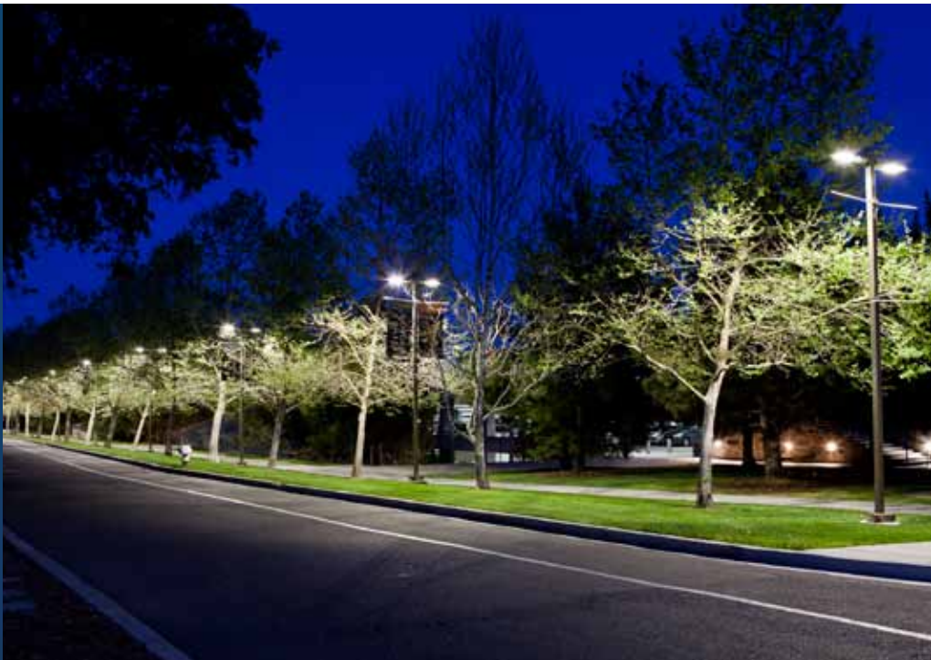
Network-controlled adaptive LED fixtures line Old Davis Road on the UC Davis campus.
