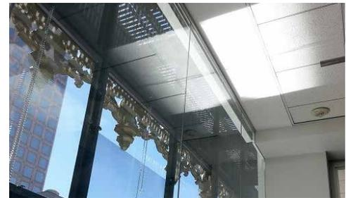
FIGURE 48 Photograph of space with light redirecting film installed at the upper area of one window pane, showing the sun shape on the ceiling from the redirection of direct solar radiation.
