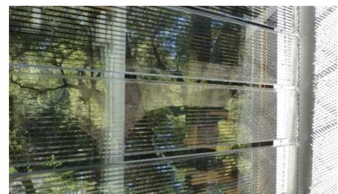
FIGURE 49 Photograph of light redirecting microstructure installed on a window, showing the direct and redirected patterns on the transmitted radiation on the side wall of the space.
