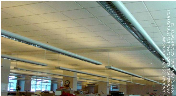
**FIGURE 63** Photograph of an open office showing electric lighting luminaires laid out in groups parallel to the window wall and controlled individually to different dimming levels based on their distance from the window walls.
