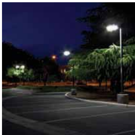
A bi-level, cobra-head induction fixture tested at the UC Davis campus continues to show potential.
