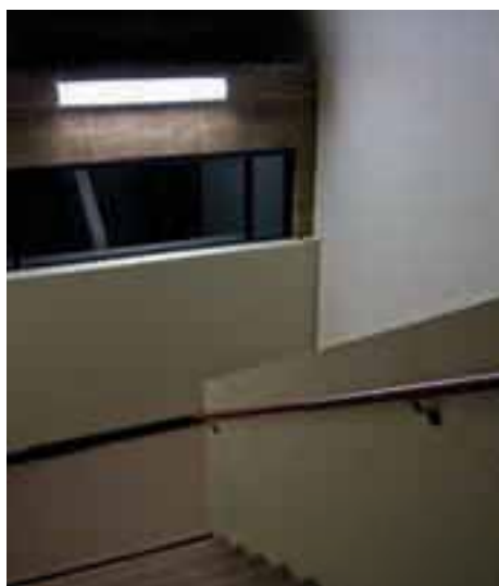
Tested at California college campuses, bi-level stairwell luminaires operate at 58 watts in high mode and 29 watts in low mode.
