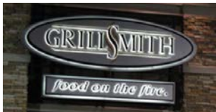
Internally illuminated sign
