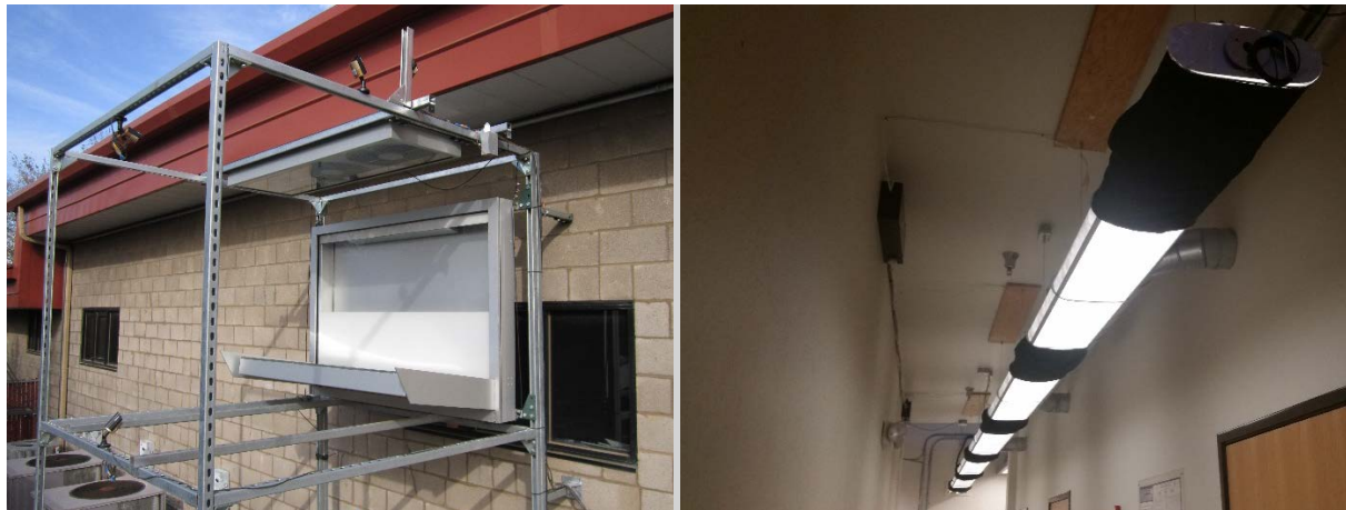
Figure 13: Core Daylighting System Installed at the CLTC
