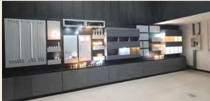
Figure 6. Lighting system wall (under construction) for education and training.
