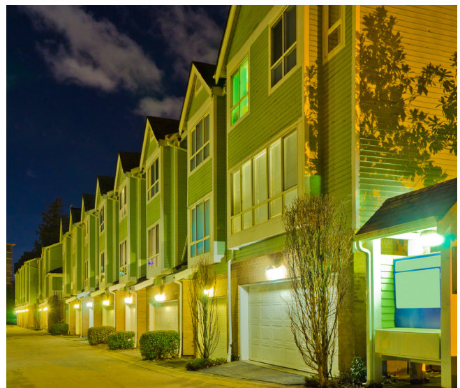
High-Rise Outdoor Lighting Controlled from Inside the Dwelling Unit
