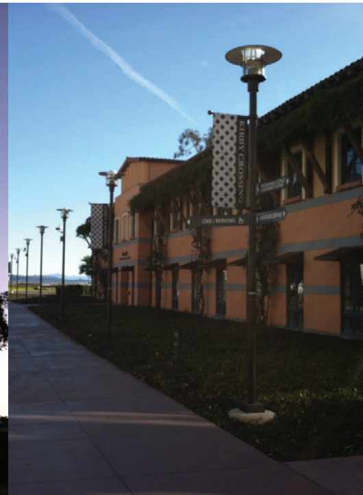
Post-retrofit network controlled LED streetlights (left) and post-top fixtures (right) at UC Santa Barbara
